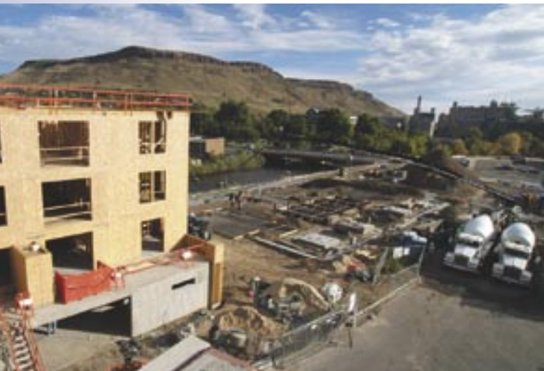
Millstone buildings one and two under construction
